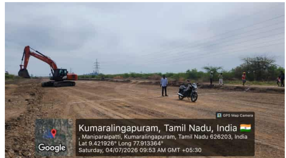
R1- C7-1+745 Culvert Excavation
