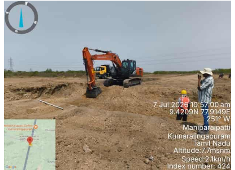
R-18 C35 0+153 -Culvert Excavation work
