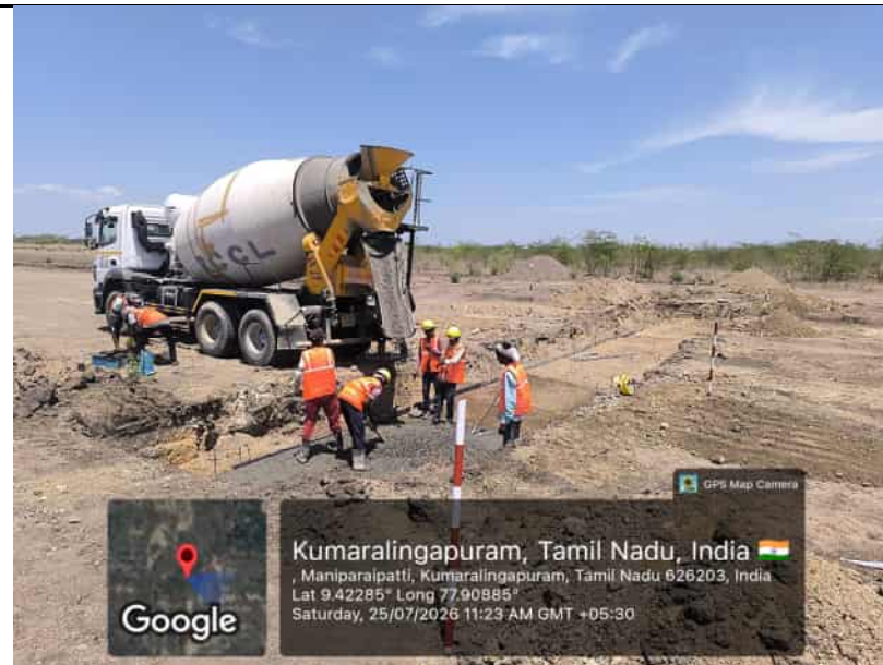
R-2 C-10 0+400 PCC Laying work
