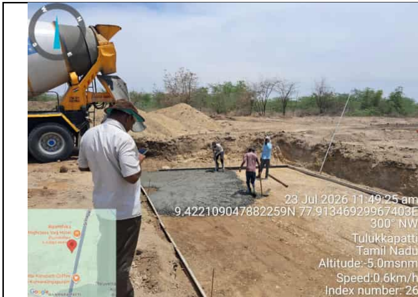
R-1 C-7 1+745 PCC Laying work
