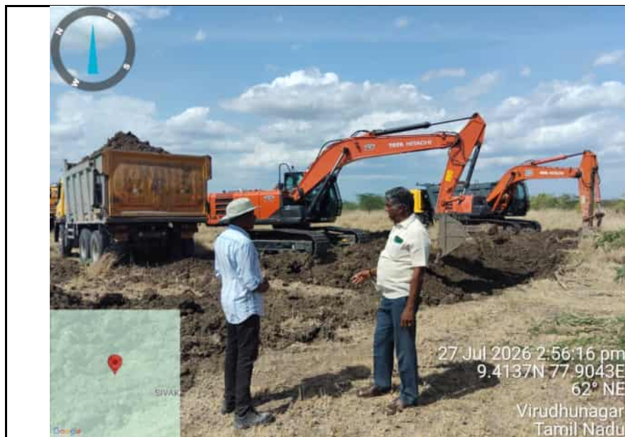
OSR-25 Top black Soil Removal work
