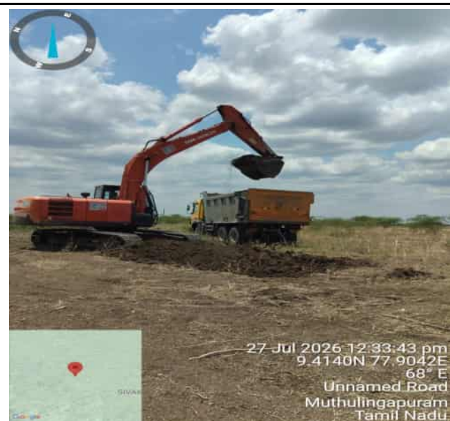
OSR-25 Top black Soil Removal work
