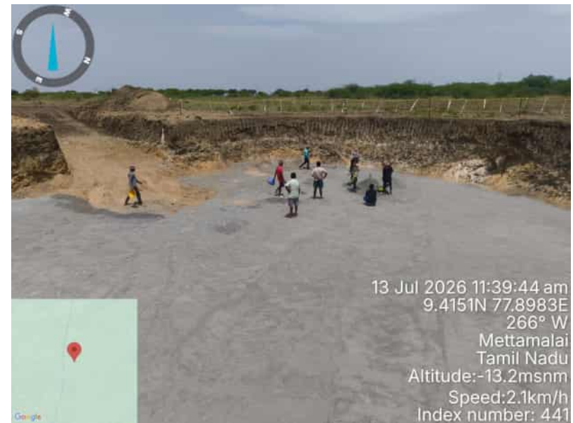
AM-6 F-ELSR-1 PCC Bed Sand Filling Work
