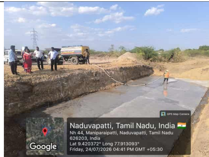
PO & EE Maam Inspection R-1 C-7 1+745 PCC
