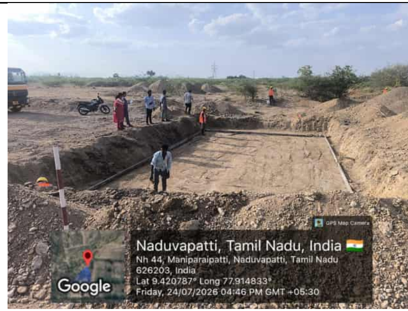
PO & EE Maam Inspection R-18 C35 0+153 PCC Bed preparation
