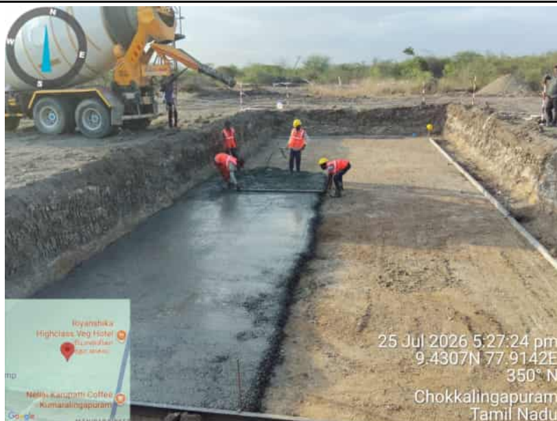
R-16 C-31 PCC Laying work
