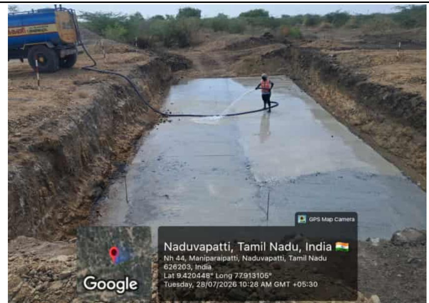
R-1 1+945 PCC Curing Work
