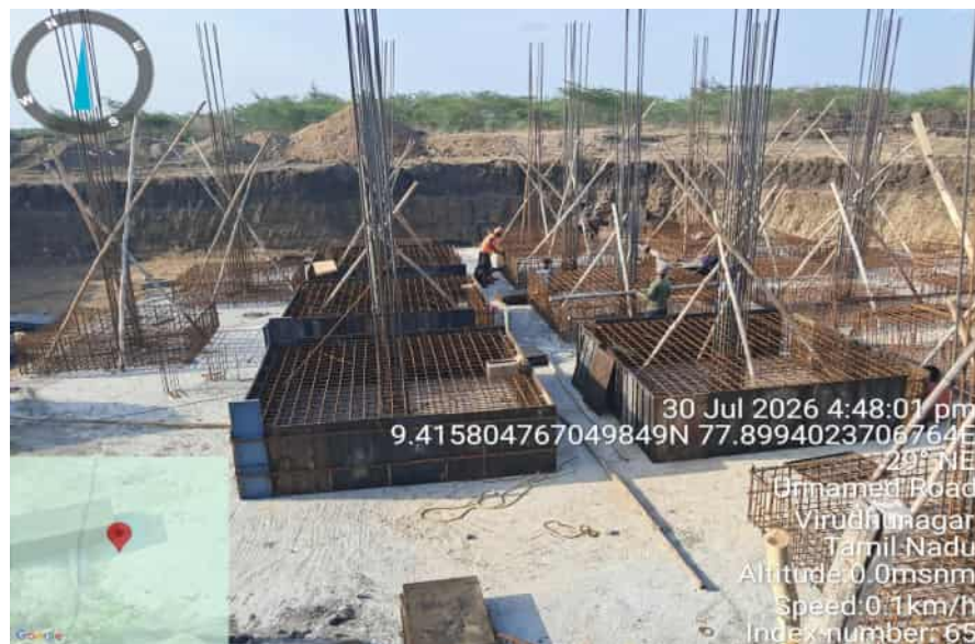
AM-6 D-ELSR-1 Footing Shuttering work
