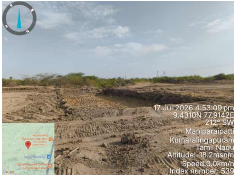
R-16 C31 0+054 Culvert EW completed
