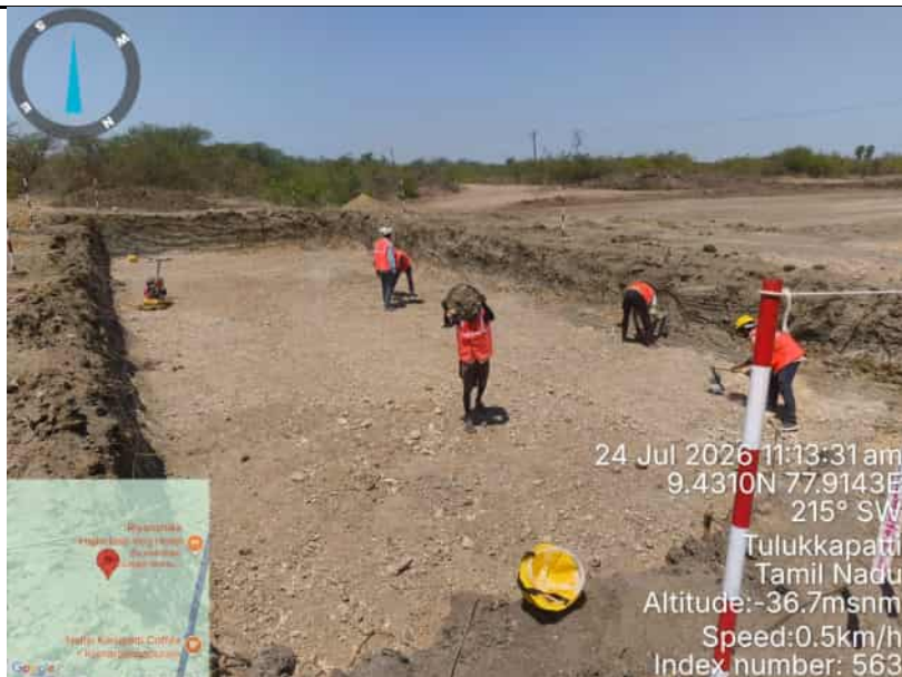
R-16 C-31 0+054 Culvert PCC Bed preparation
