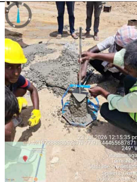
Slump Cone Casted Work
