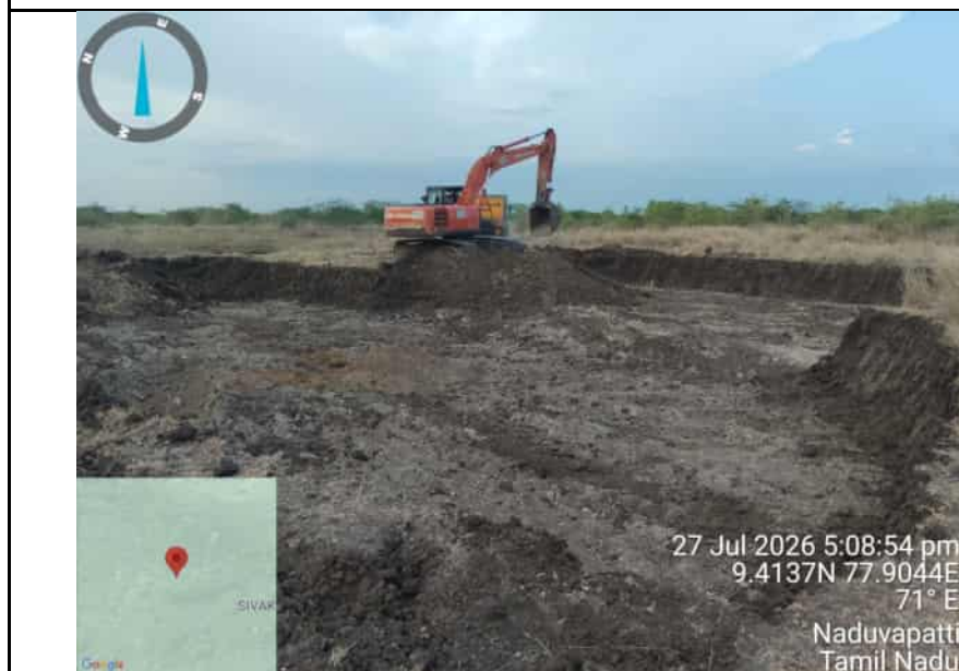
OSR-25 Top black Soil Removal work
