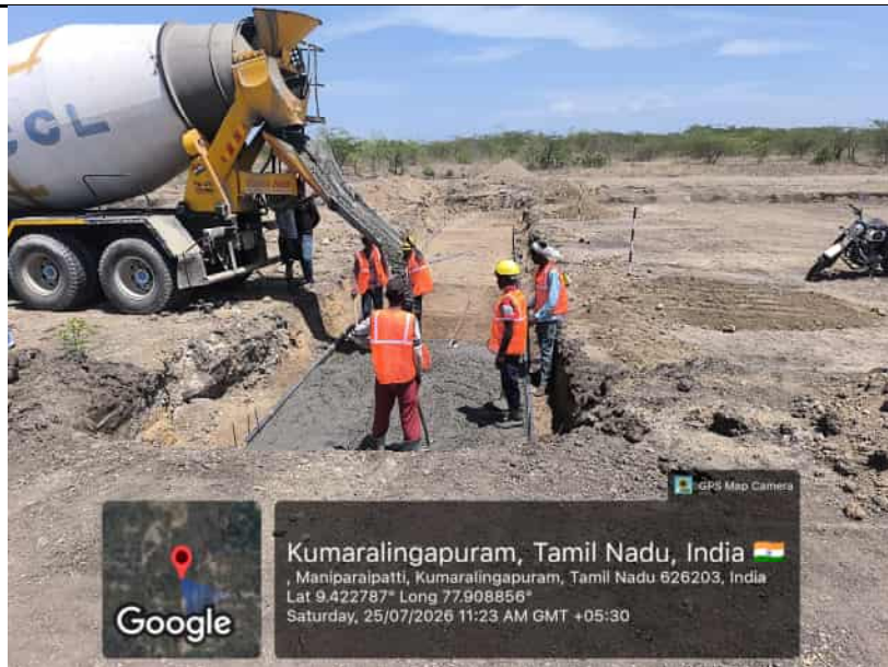
R-2 C-10 0+400 PCC Laying work
