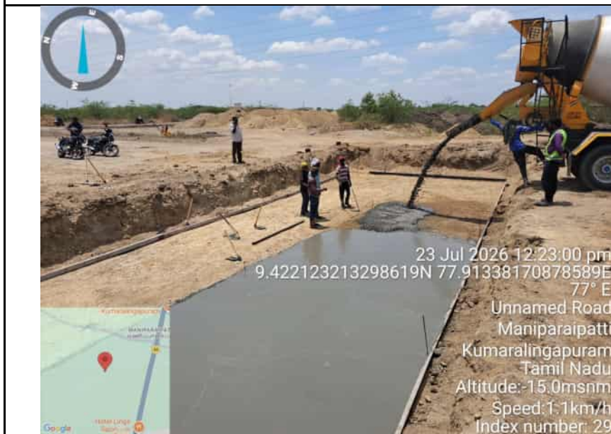
R-1 C-7 1+745 PCC Laying work
