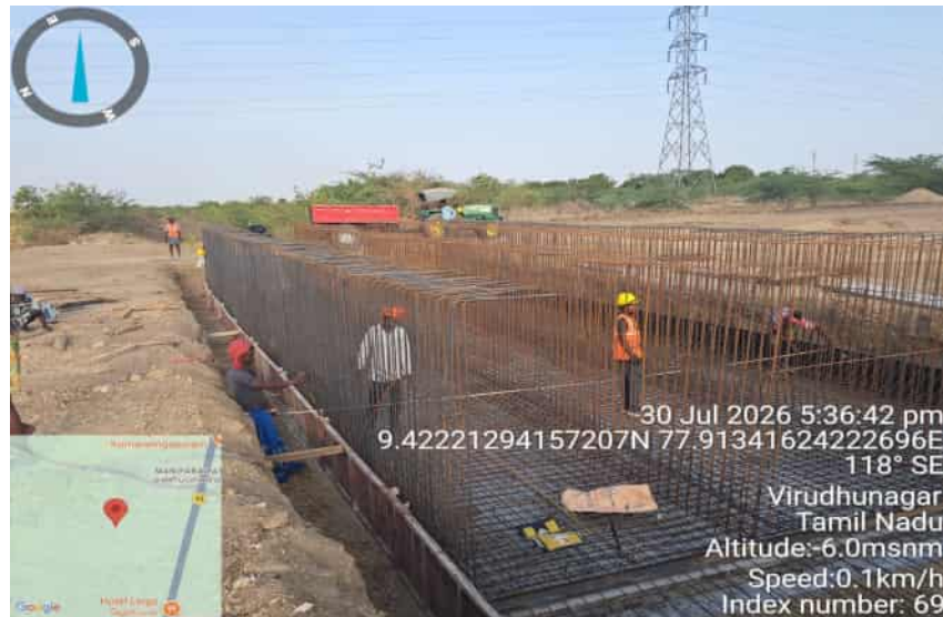
R-1 1+745 C-7 Culvert Reinforcement Work
