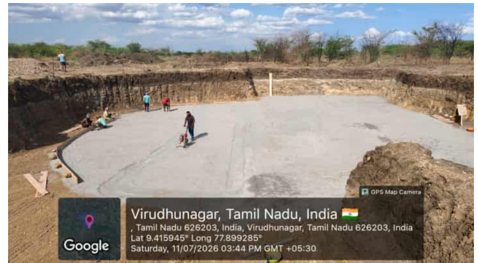
M-6 D-ELSR-1 PCC Bed Preparation & Compaction work
