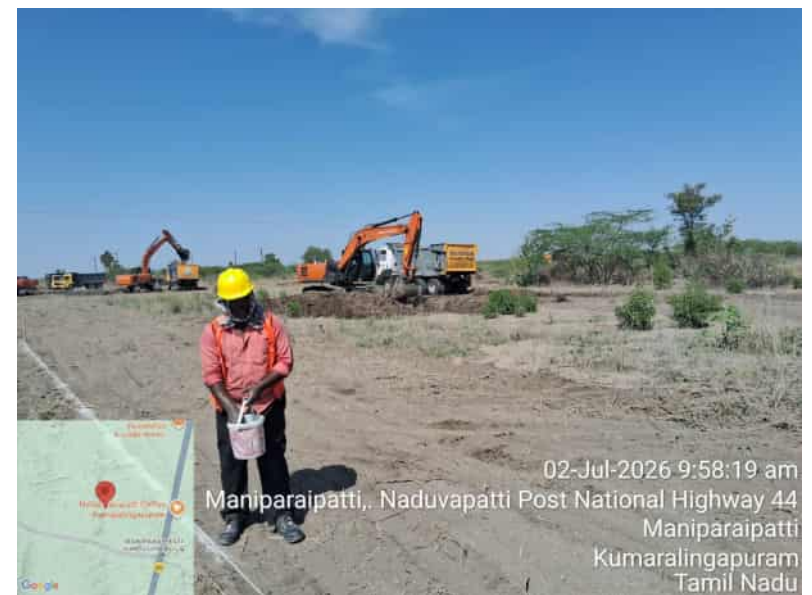
Road NO-1,Outer line marking
