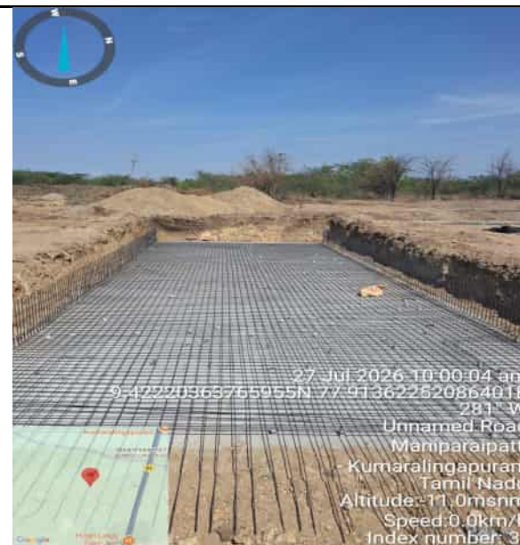
R-1 C7 1+745 Raft Reinforcement Tying
