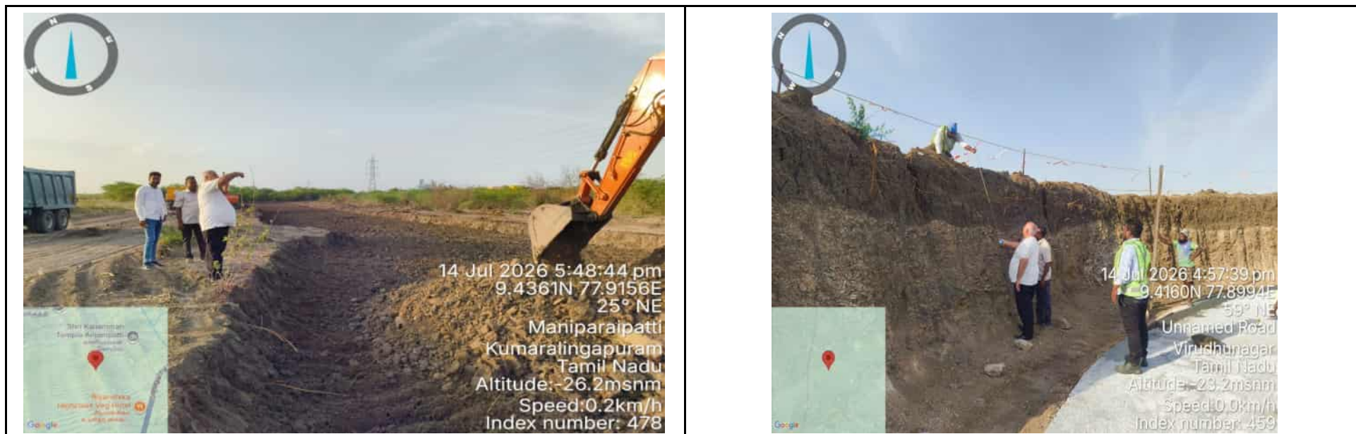
PD Inspection at D-ELSR black soil depth checking
