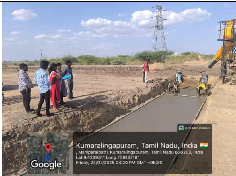
PO & EE Maam Inspection R-1 C-6 1+563 PCC Laying
