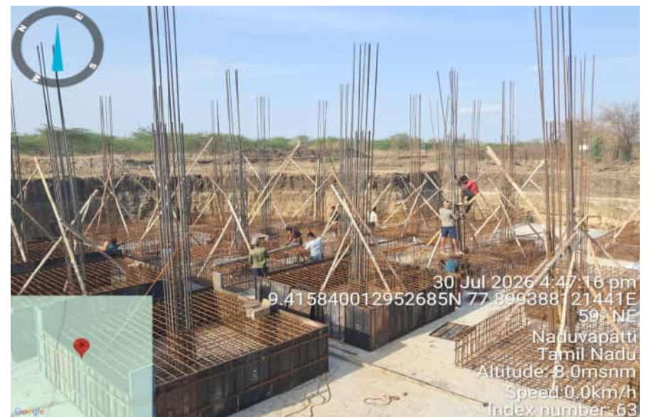
AM-6 D-ELSR-1 Footing Shuttering work
