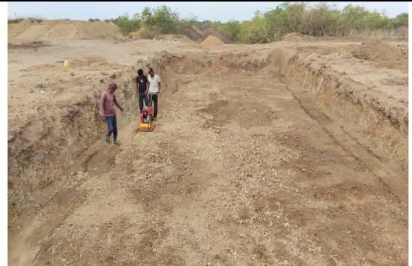
Road No-1 C-8 0+945 Culvert pcc Bottom Section work.
