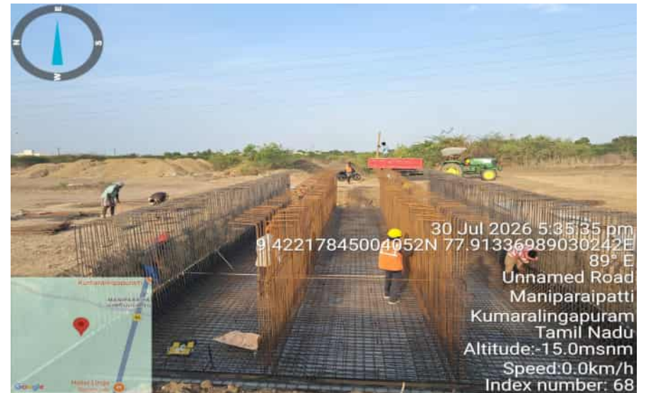
R-1 1+745 C-7 Culvert Reinforcement Work
