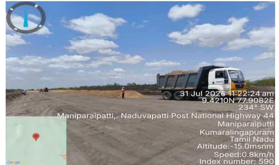
R-2 Embankment Soil Dumping
