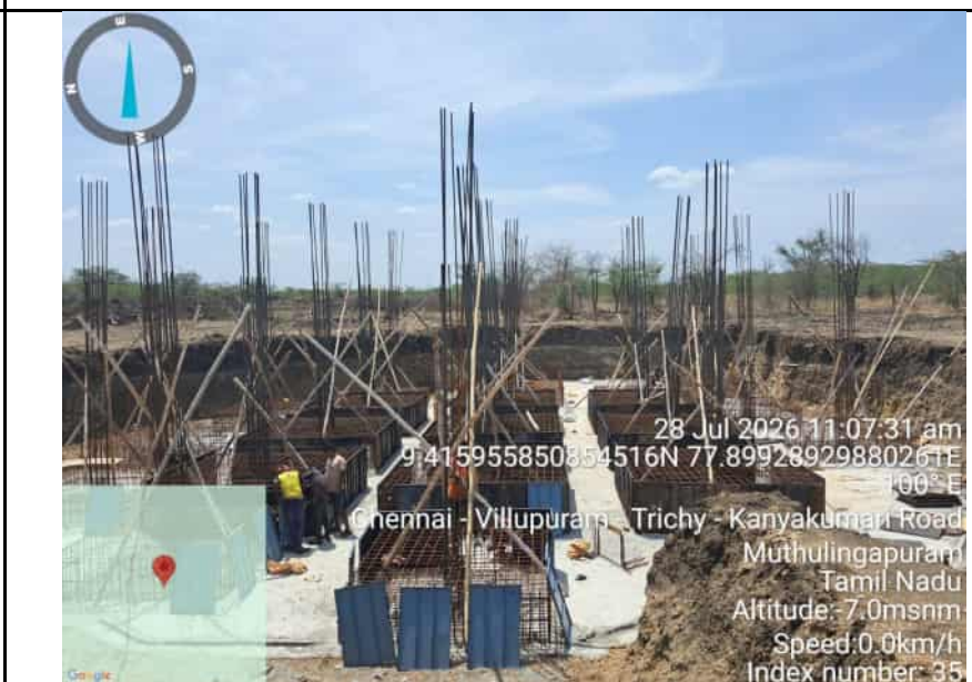
AM-6 D-ELSR-1 Footing Tying & Shuttering work
