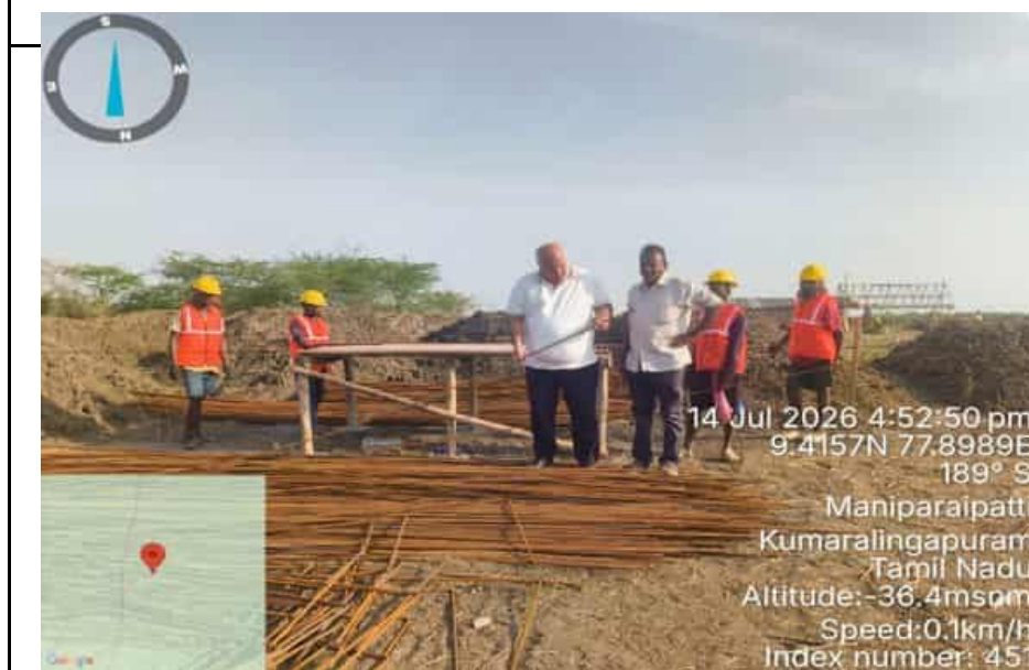
PD Inspection at R-1 Road CNG Work
