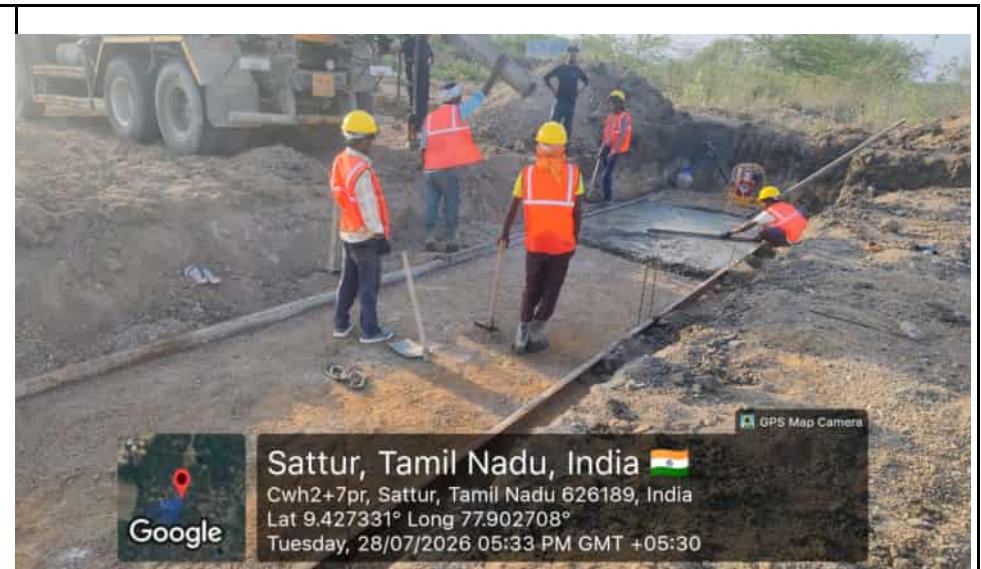
R-20 C38 PCC Laying work
