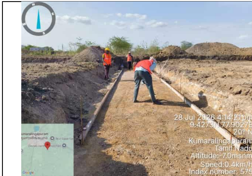
R-20 C38 PCC Side Shuttering Work
