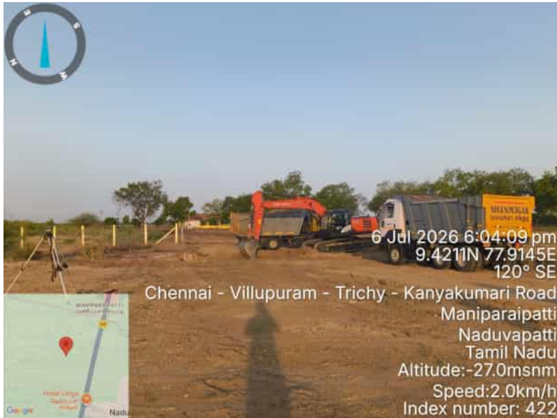
R-18 C35 0+153 -Culvert Excavation work
