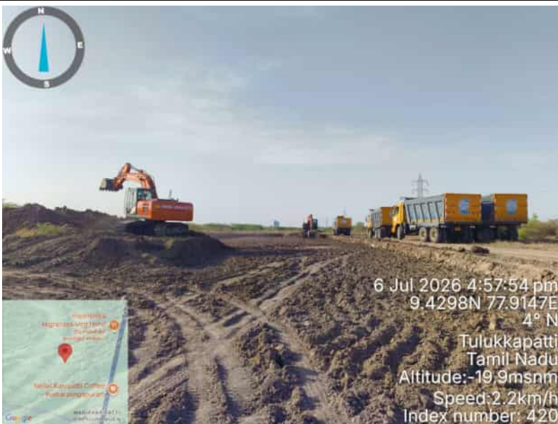
Road NO-1,CNG Work
