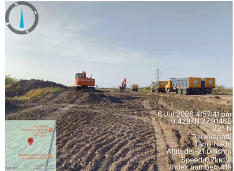
Road NO-1,CNG Work
